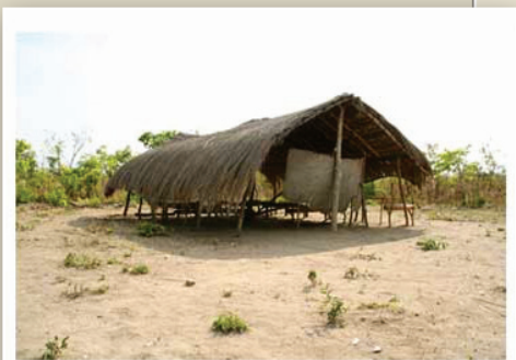
Many communities don't even have a school like this.
